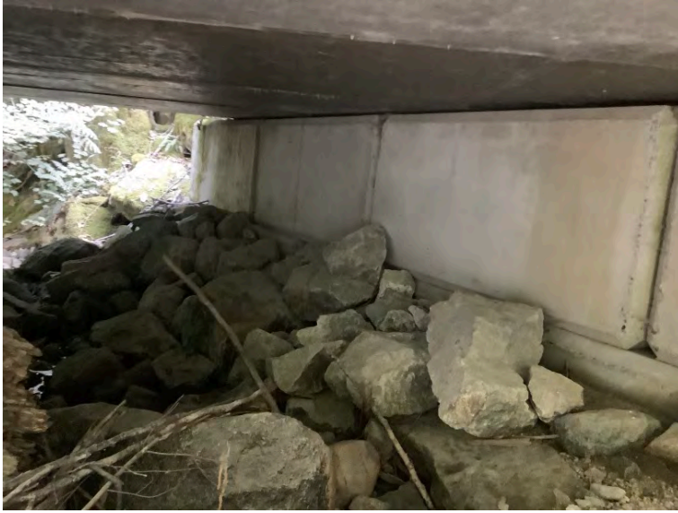
Right Bank Abutment when facing downstream
