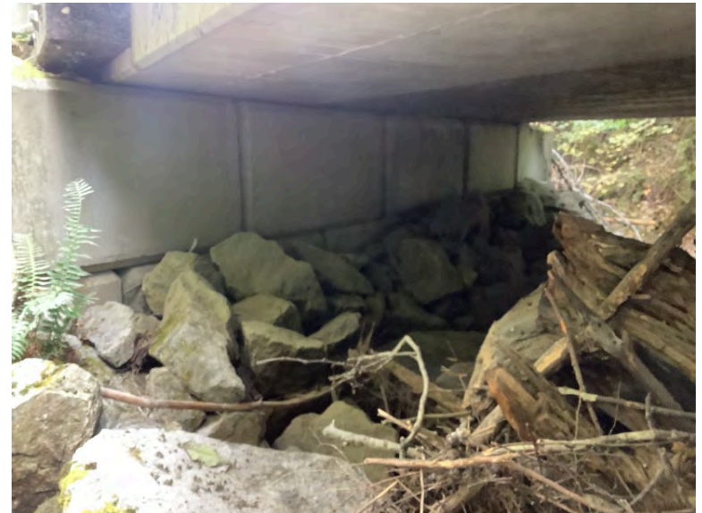
Left Bank Abutment when facing downstream
